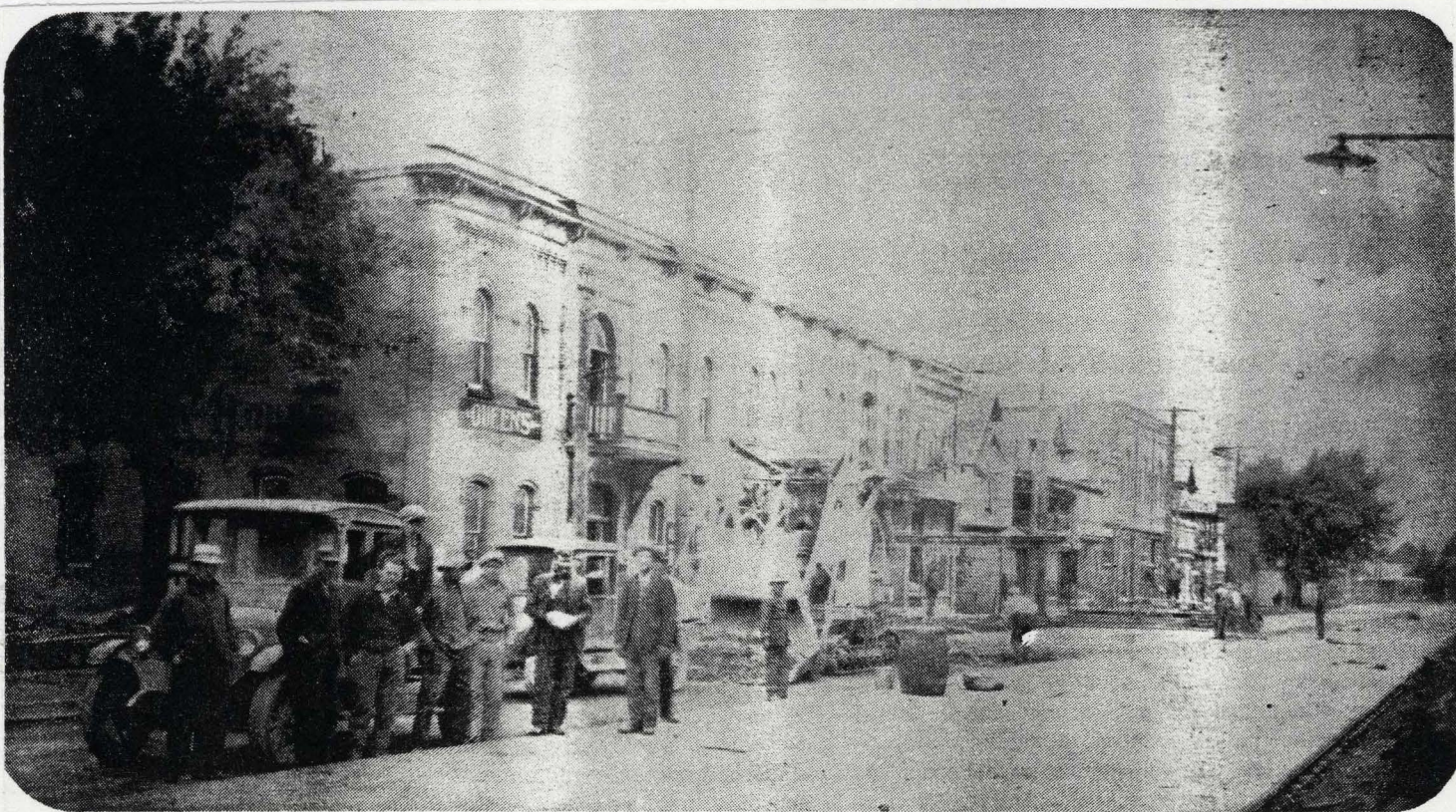
Paving Furnival in Rodney's business section in 1928
