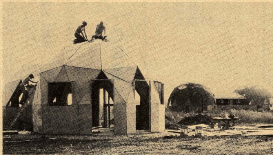
DORMITORIES ARE BEING BUILT AT TWIN VALLEYS SCHOOL by students using the same geodesic design for the roof as in the original classroom living quarters in the background.
